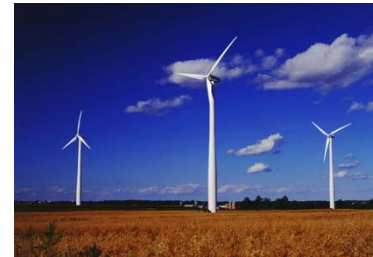
Distributed generation grid connections
