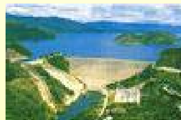
Kwae Noi Dam 30.0 MW
