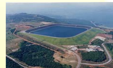
Lam Takong Pumped Storage 500 MW
