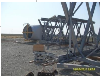
Azerbaijan ( Wind Tower 160 m high)
